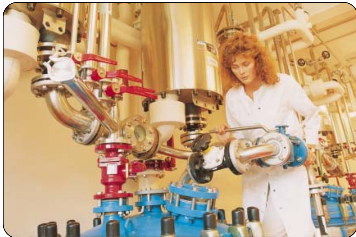
Vent piping for pharmaceutical manufacturing in 654 SMO®
